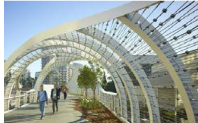
02 Footbridge (Rainbow bridge, USA)
