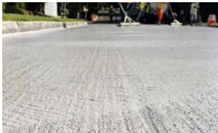
Asphalt cooling spray application
