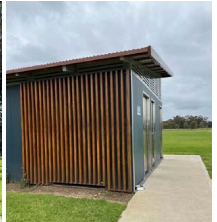
4 Recent, high quality toilet block amenity, installed in the southern half of the park.
