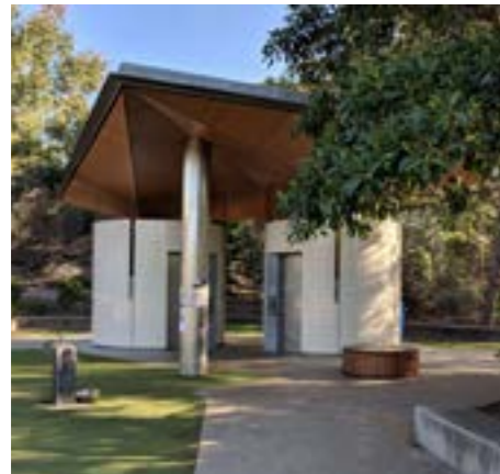
Shade structure with toilet facilities and storage
